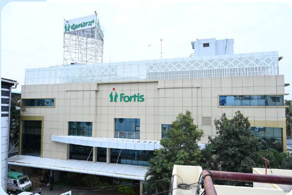
Fortis Hospital, Nagarbhavi
